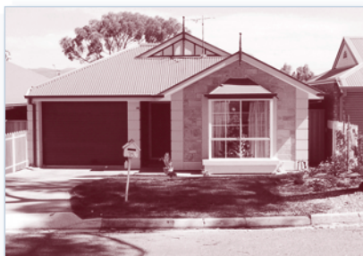
1998: Three bedroom housing constructed by the Trust at Holden Hill.
