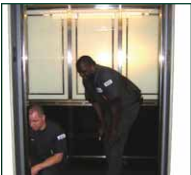
Building engineers make their final inspections of the first modernized elevator prior to its release for service.
