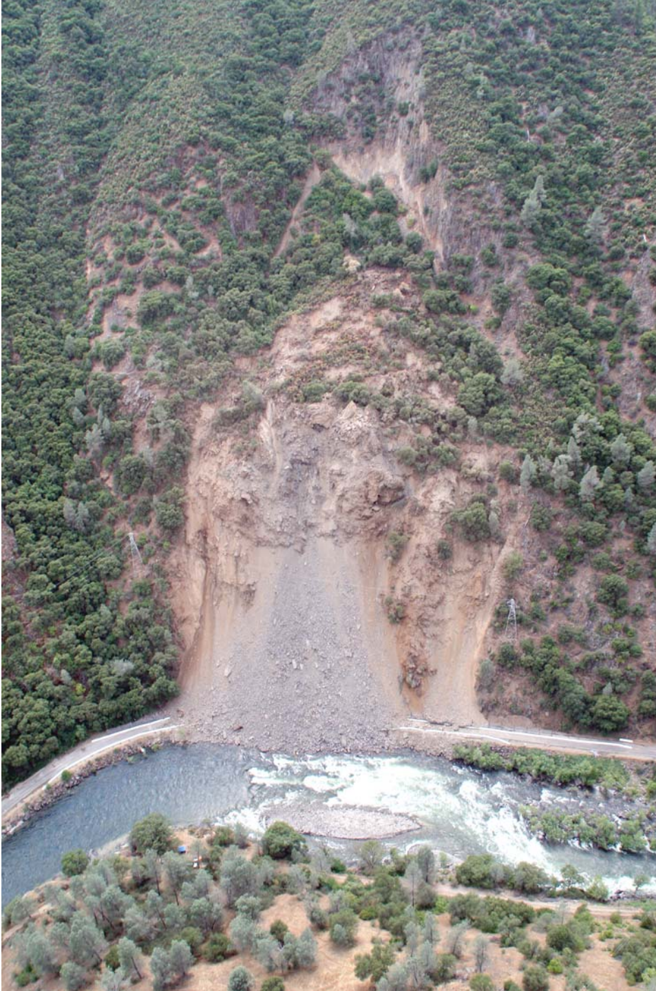
Figure 1. Oblique aerial photograph of Ferguson Rock Slide. Merced River in foreground is flowing left to right. Photo taken by Ed Harp, USGS on June 13 th , 2006.
