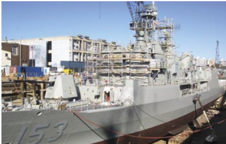
HMAS STUART undergoing refit at ADI's Garden Island Facility.
