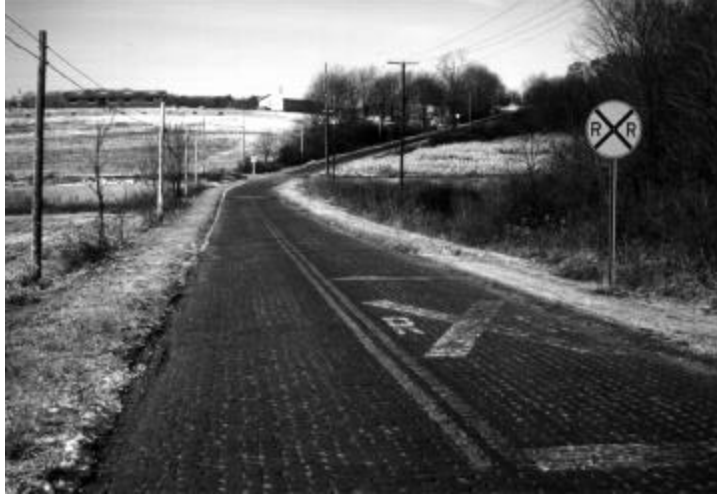
Bypassed by a second generation Lincoln Highway, Stark County's Baywood Street brick section preserves the 1920s pavement of the original road. (Kevin Patrick)
