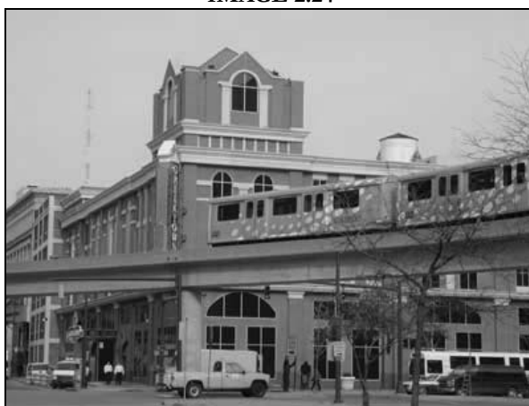
Detroit’s Greektown casino is rare in its location adjacent to a rail transit station.
