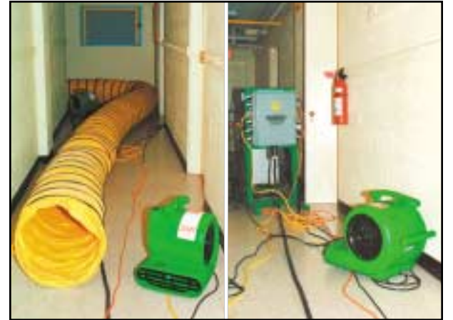
Above: A 5000-cfm desiccant dehumidifier utilized by Servpro, along with two diesel generators, power distribution equipment, and carpet dryers, to dry out a flooded basement at St. Lukes Episcopal Church in Norfolk Below: Inside views of the church basement during restoration
