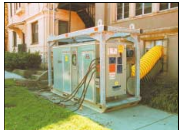
Above: A 5000-cfm desiccant dehumidifier utilized by Servpro, along with two diesel generators, power distribution equipment, and carpet dryers, to dry out a flooded basement at St. Lukes Episcopal Church in Norfolk Below: Inside views of the church basement during restoration
