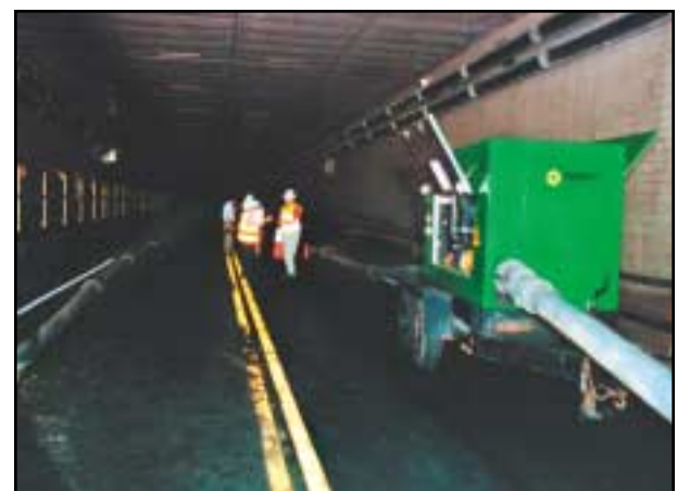
Above: A 375-cfm diesel air compressor rented by Garner Environmental Services to power venturi air horns providing ventilation inside the flooded Midtown Tunnel in Norfolk Below: One of two 6" Quiet Flow™ pumps utilized by Garner Environmental inside the Midtown Tunnel
