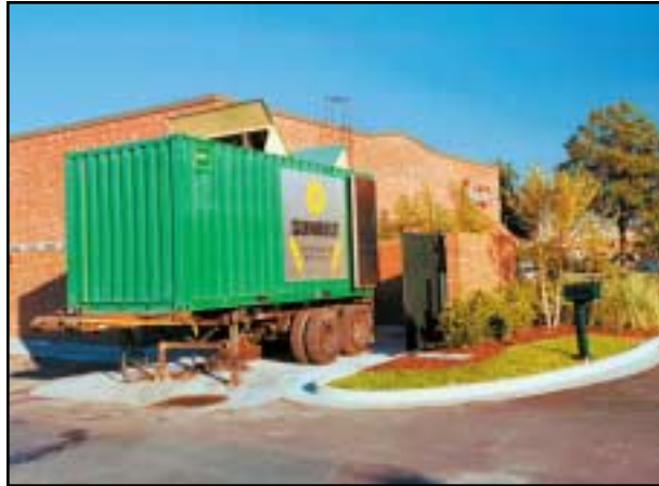
Above: A 500-kW diesel generator provided emergency power for the USS Kauffman at Colonna's Shipyard in Norfolk. The ship was moved to the Navy Yard for safekeeping during Isabel. Below: A 350-kW generator powering an O'Charley's restaurant in Richmond during power outages
