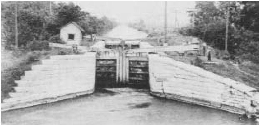
Locks on the Illinois and Michigan Canal at Marseilles.
