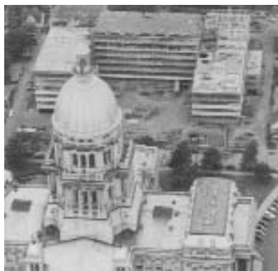
Construction of the Stratton building, west of the Capitol, began in 1954.
