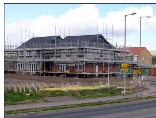
Greenfield Release Housing Construction - Drumchapel
