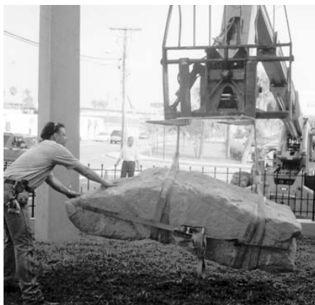
Installing the 3,000 pound rock.
