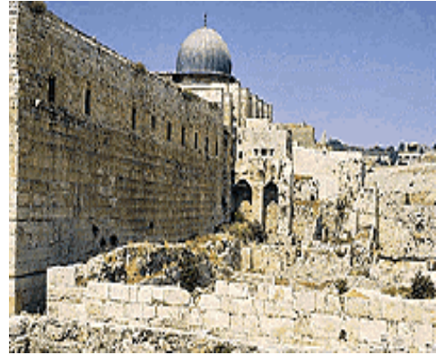
Jerusalem showing water baths and water carrying structures
