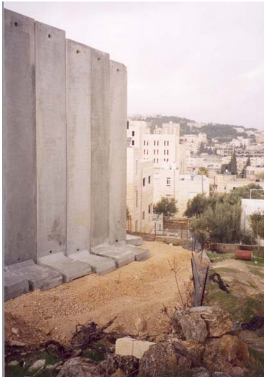
The Wall in Abu Dis January 2004
