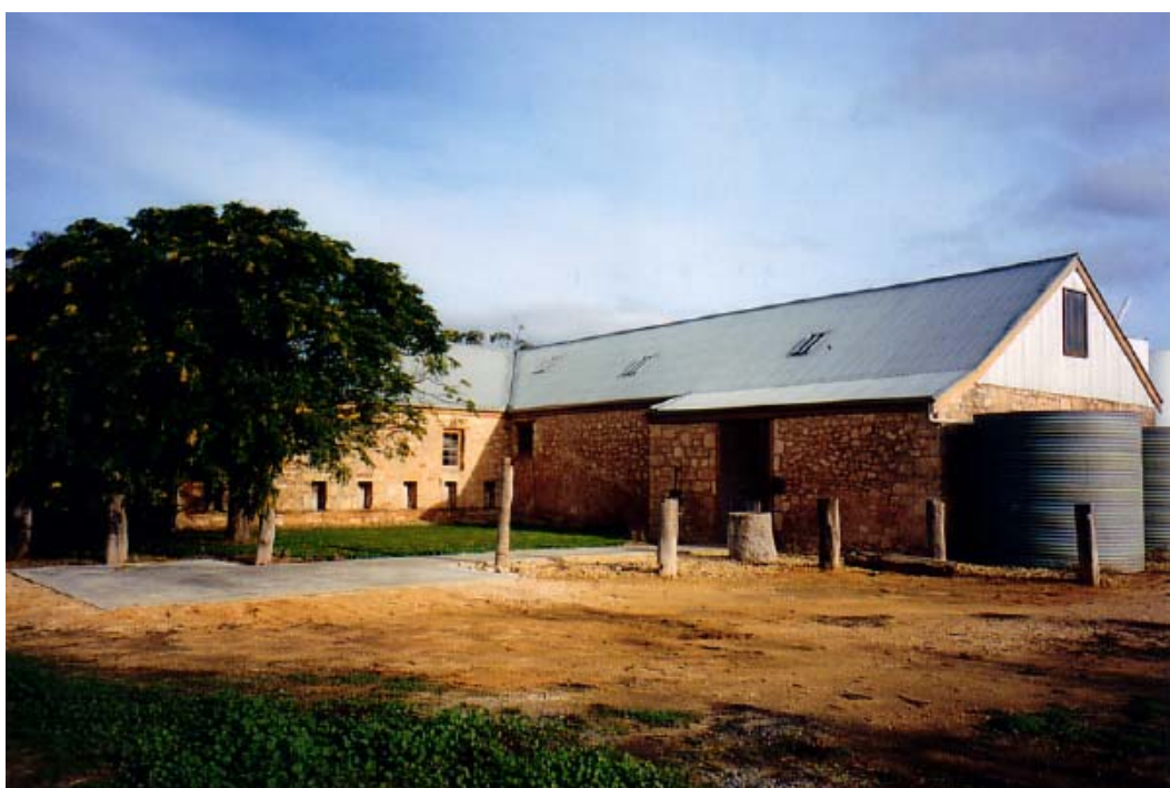
Padthaway shearing shed, looking south
