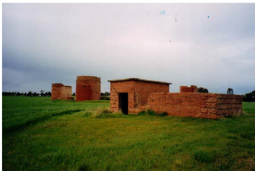
Wolseley IAFD, pump house and 1941 fuel tanks
