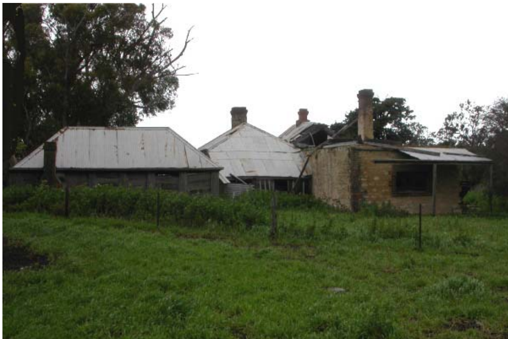
Charla Homestead, slab kitchen at left
