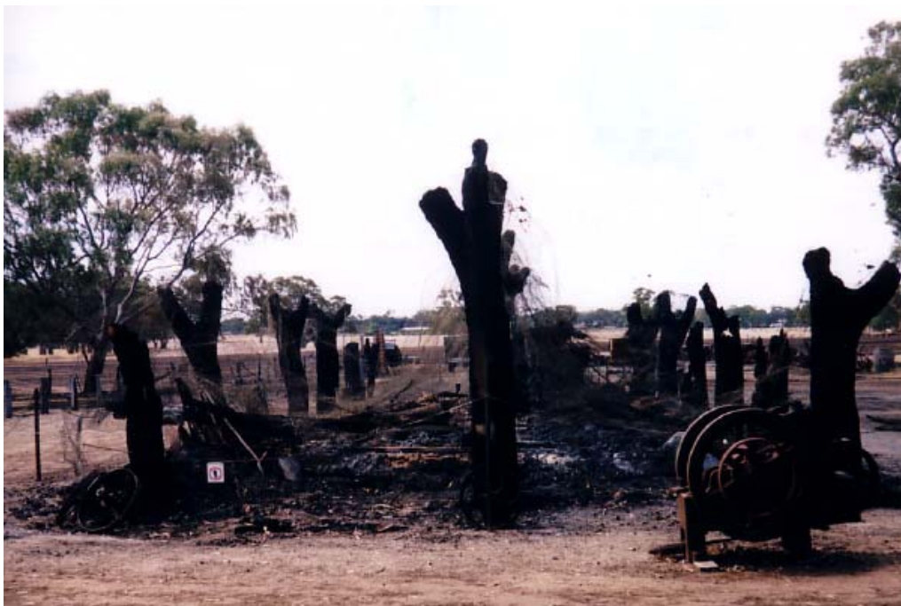
Clayton Farm silage pits after fire, looking north
