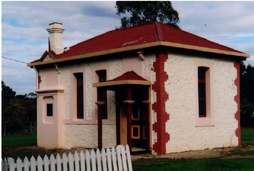
Wirrega Council Chambers, looking south
