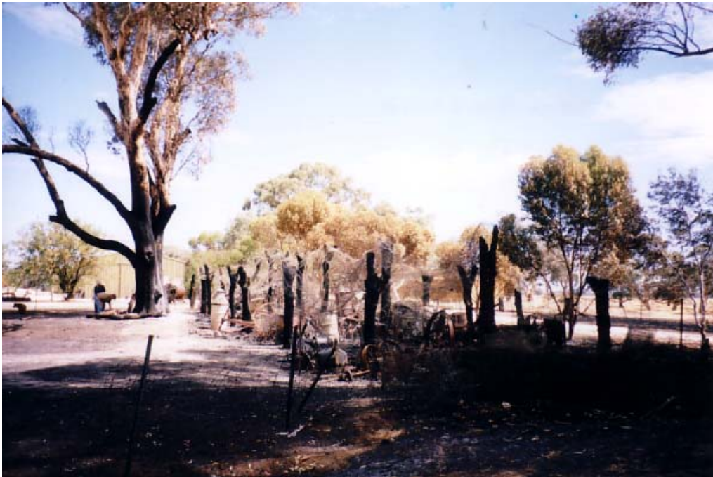
Clayton Farm buggy shed after fire, looking south-west
