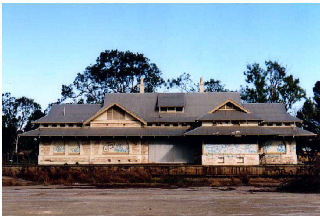
Bordertown Railway Station, looking south-west
