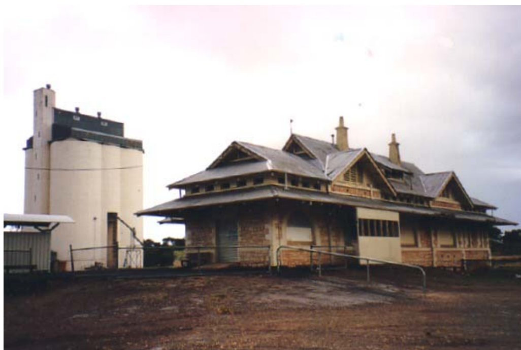
Bordertown Railway Station, looking east
