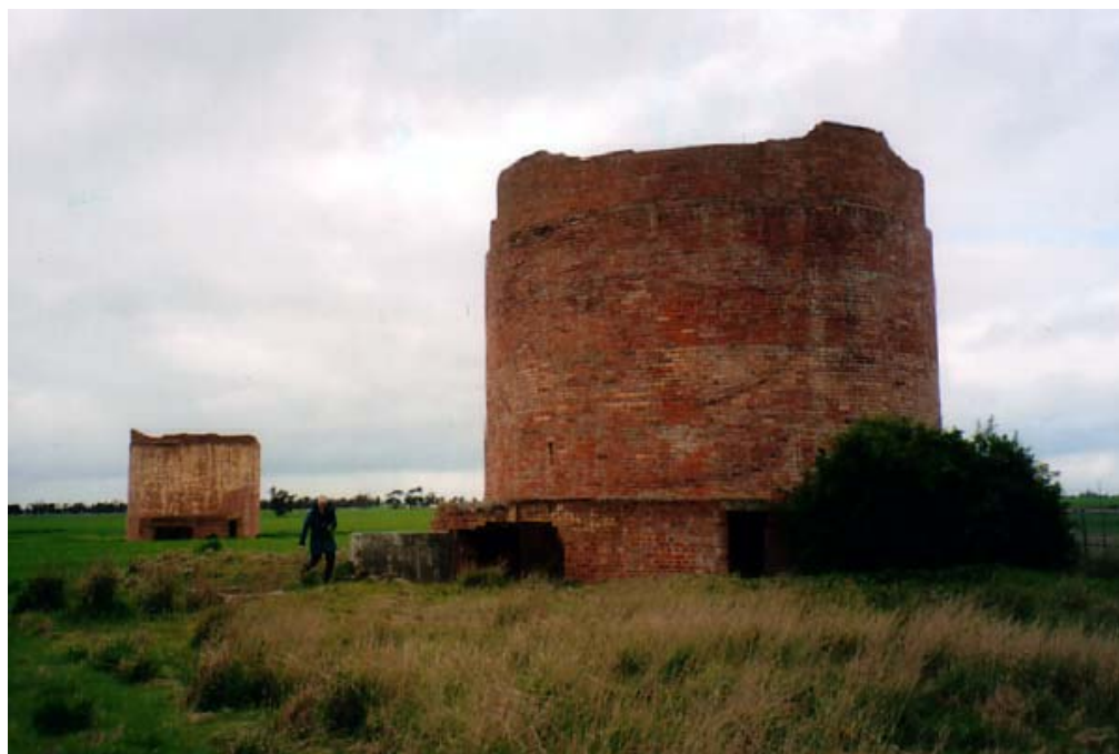
Wolseley IAFD, brick fuel tanks (1941)
