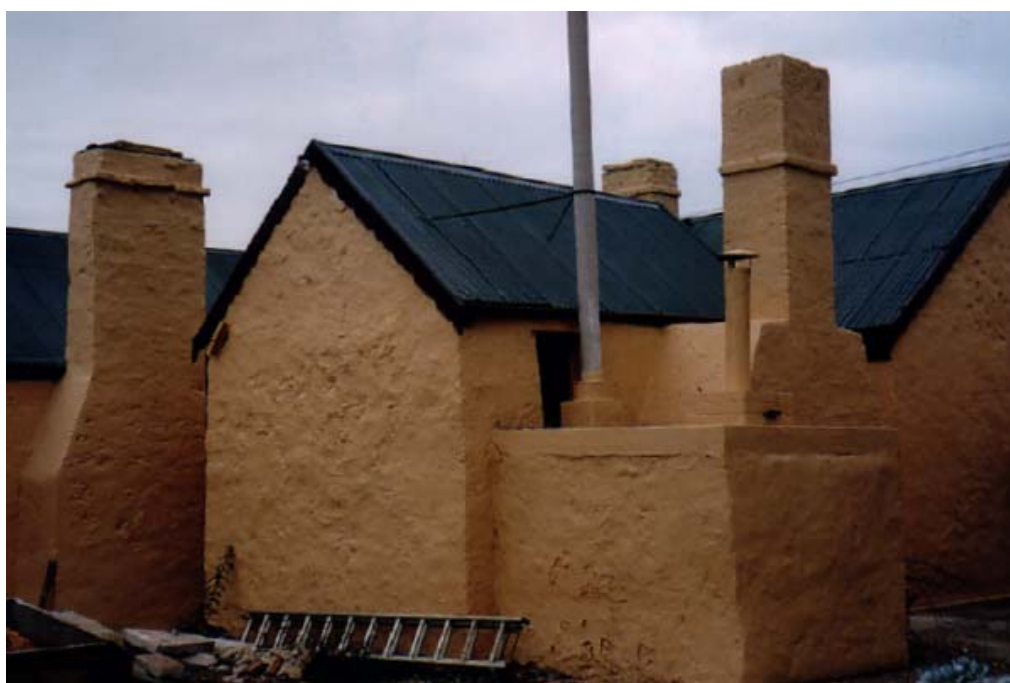
Mundulla Hotel Kitchen, looking south-west
