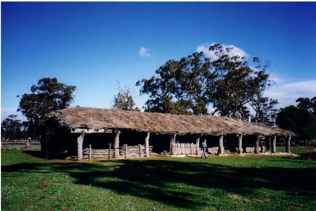
Clayton Farm woolshed, looking south
