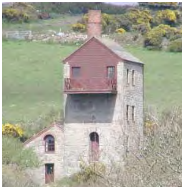
Wheal Enys, Porkellis. Whilst residential use is not always appropriate, this conversion has been done sympathetically.
