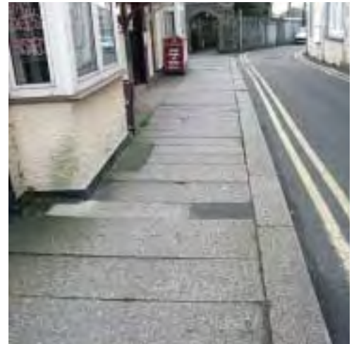
Camborne - street paving. Granite paving slabs are a distinctive element of the urban fabric in towns across Cornwall and west Devon.
