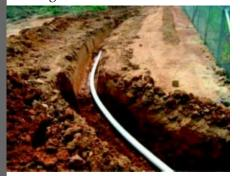
The full installation took only 12 days from the uncoiling of the first pipe until welding of the last fitting, including trenching and backfilling of the pipeline. The actual uncoiling and welding time is much less, however the civil works took the full installation time.
