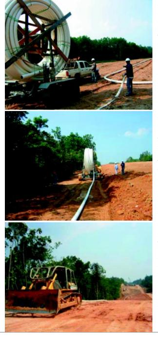
through a minor river and 7 creeks all located between large steep hills. The pipeline is installed in a 1.5-metre deep trench.
