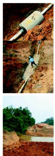
ever the uncoiling can also be performed by fixing the trailer and pulling the pipe over the RoW. In case of rocky ground wooden logs or rollers will protect the pipe for damages.
