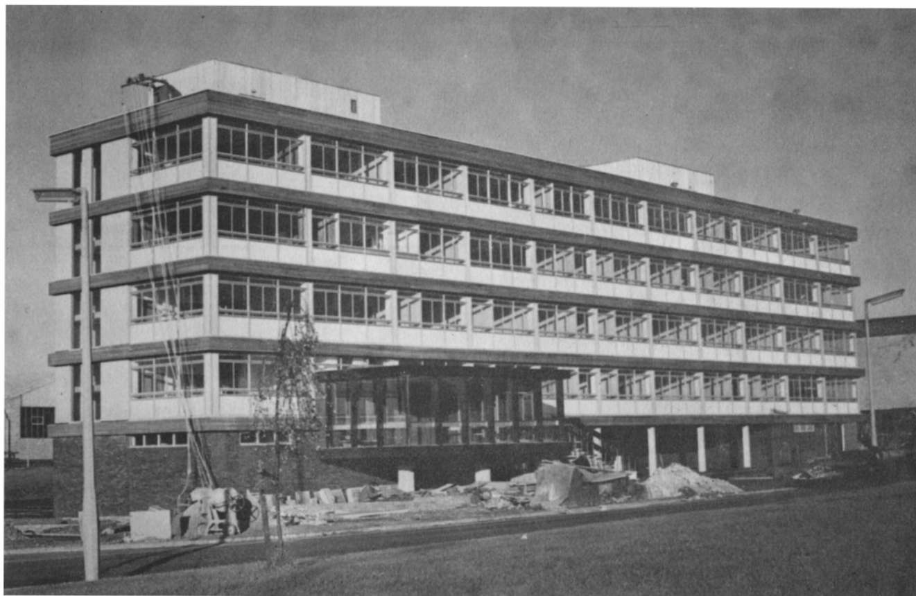
Ready for occupation: The new office block at Basingstoke
