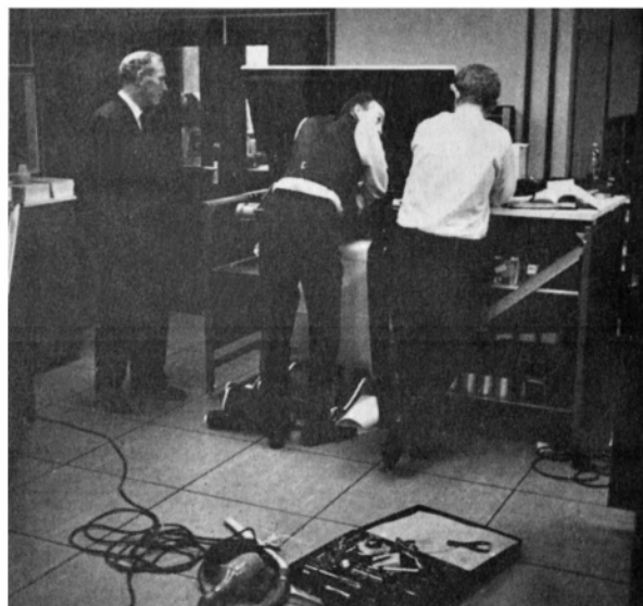
The computer being installed in its dust-proof room at Basingstoke.
