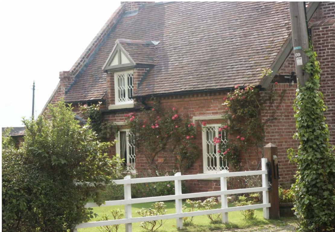
View of Vicarage Cottage
