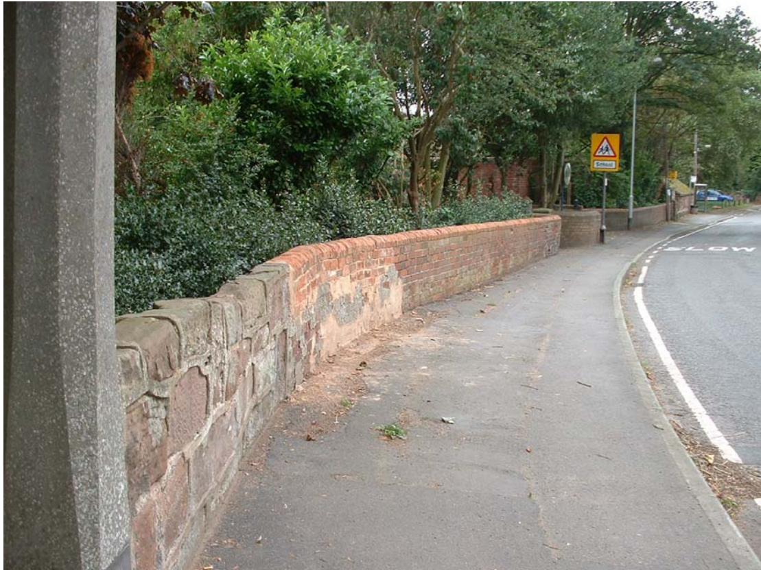
View showing a mix of sandstone and brick walls
