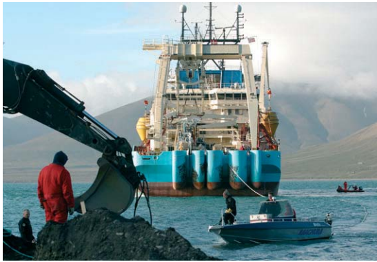
The final metres of the fibre are put in place by the cable ship on the sea floor reaching Spitzbergen in August 2003
