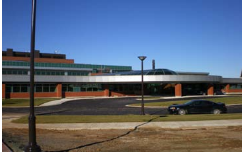
A view of the new Ambulatory Care Centre looking from Connaught Ave. The project is well underway and is expected to open in Spring 2008.
