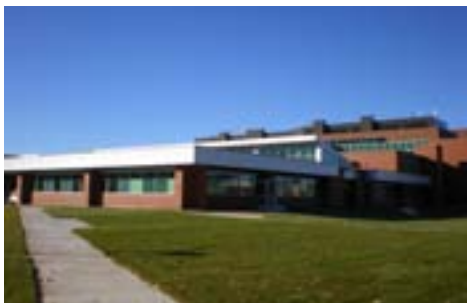
The view of the Ambulatory Care Centre from Walsh Street.
