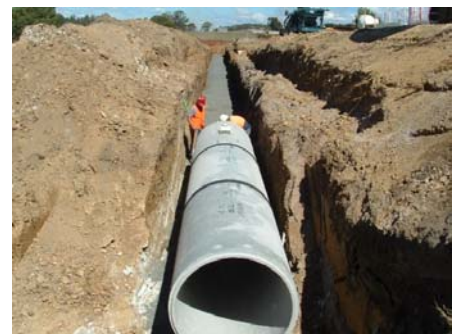
Photo 2: Lying culverts under highway
