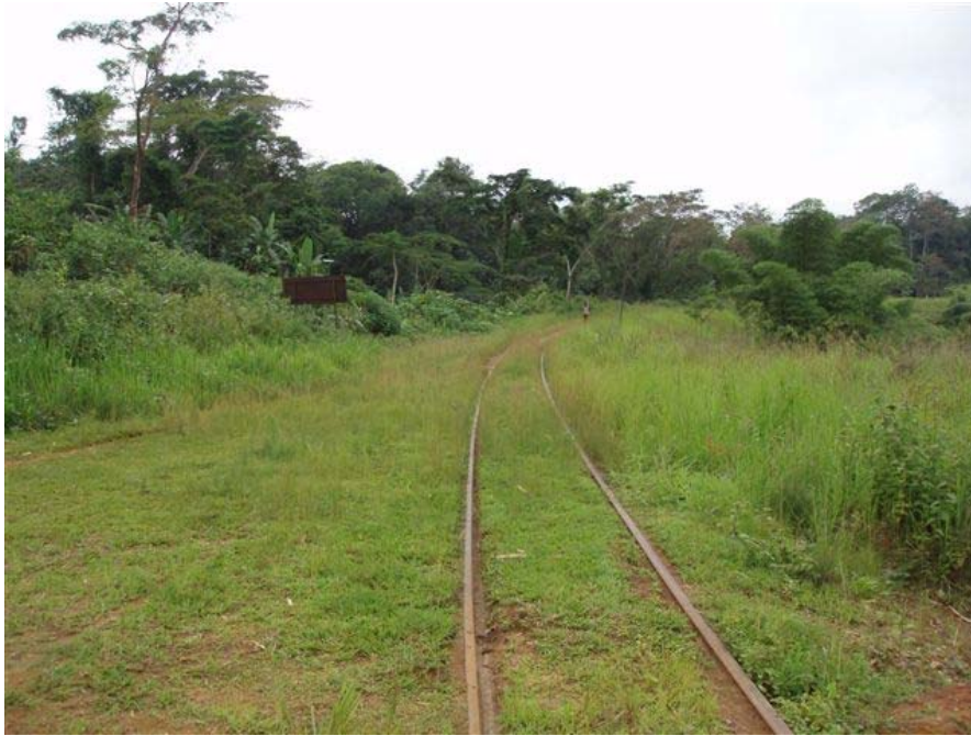
Figure 1 – Pointe Noire to Mbinda rail line
