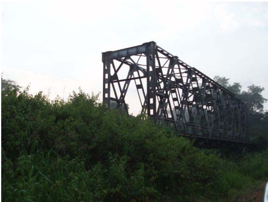
Figure 2 – Steel framed bridges on Pointe Noire to Mbinda line
