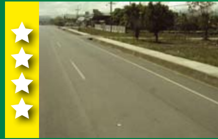
Paved sidewalk separated from traffic by a deep ditch
