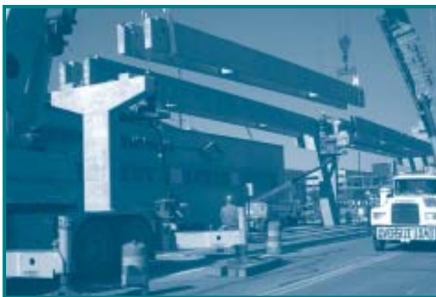
The guideway’s 173 pre-cast concrete spans range in length from 80 to 110 feet.
