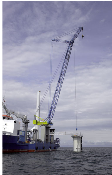
Figure 2.5: A2Sea vessel installing platform onto foundation (Courtesy of A2Sea)
