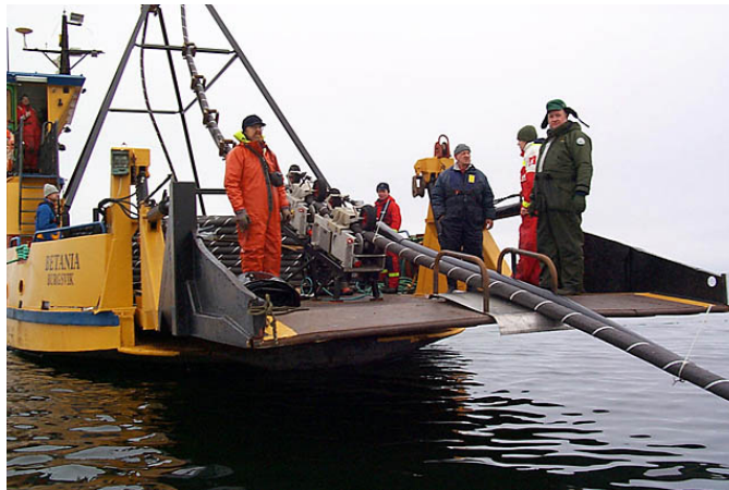
Figure 2.9: Laying cable between turbines and to shore (Courtesy of www.windpowerphotos.com )
