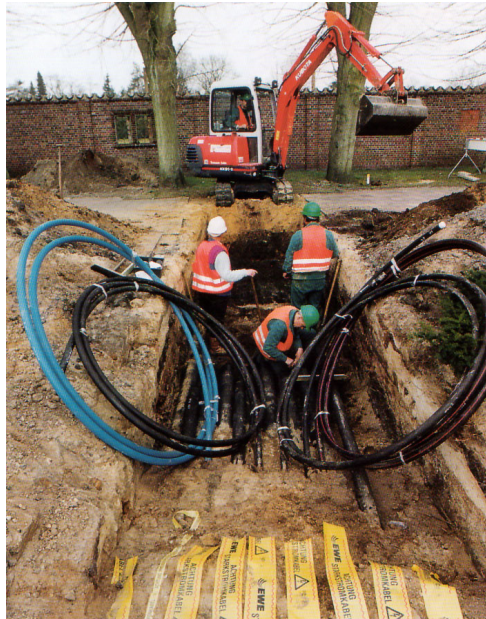
Figure 2.13: Installation of cables in a trench (Courtesy of Bohlen & Doyen)
