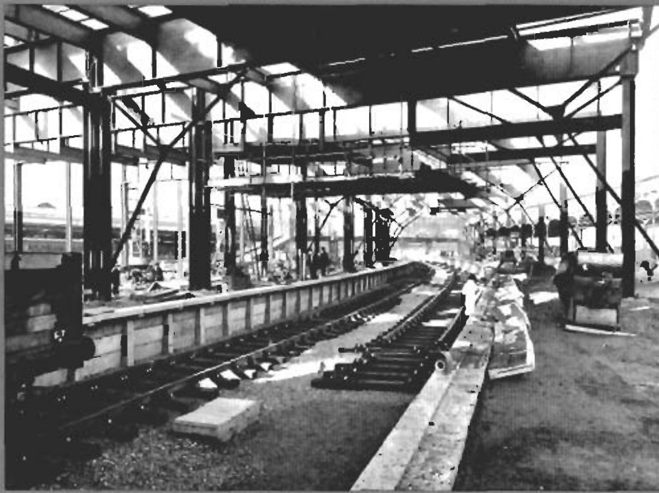
The new platforms under construction
