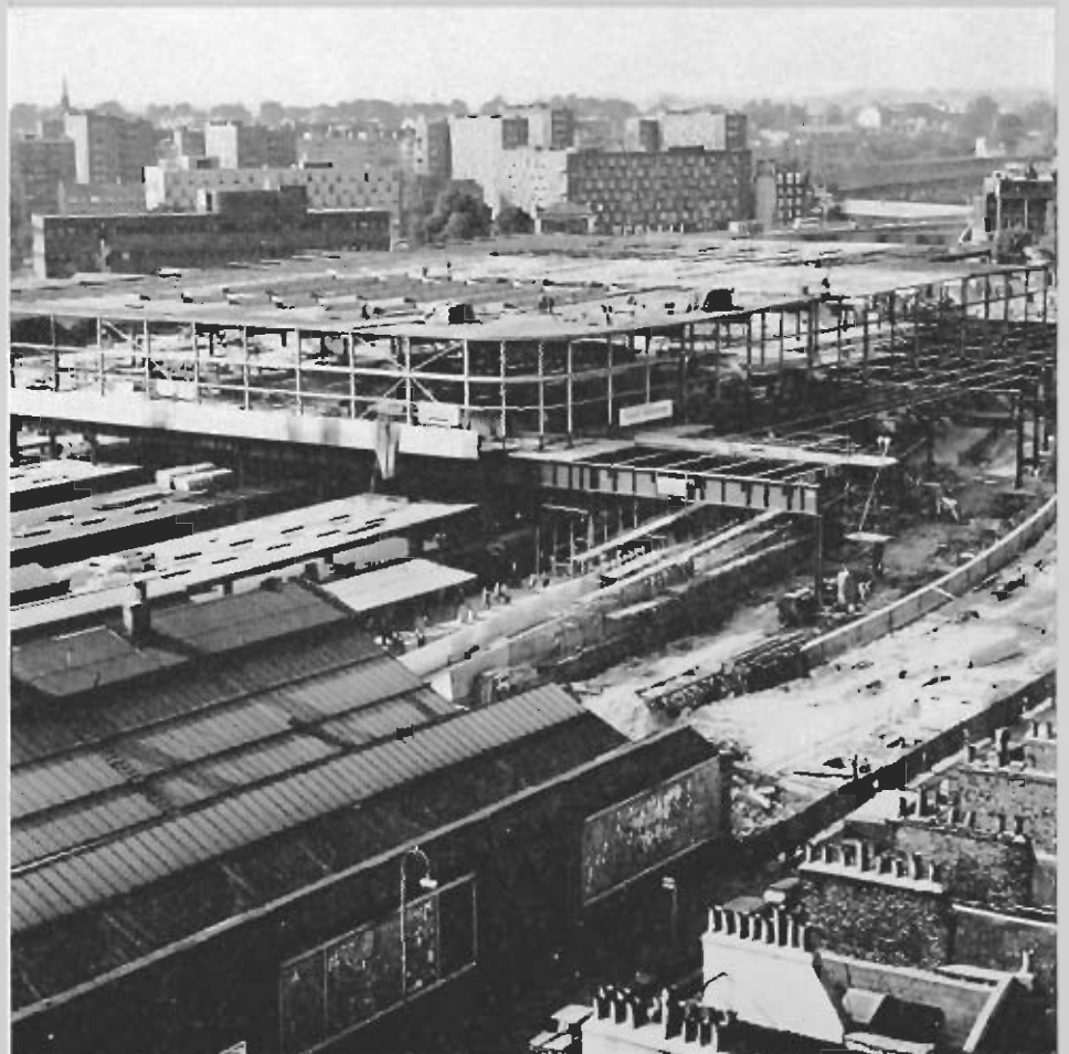
Partial construction of No. 1 platform and the parcels deck. The completed signal box and telecommunications centre can be seen in the background
