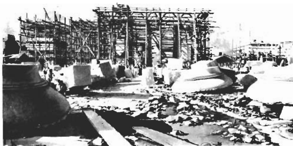
The Doric Portico at Euston under construction in 1837
