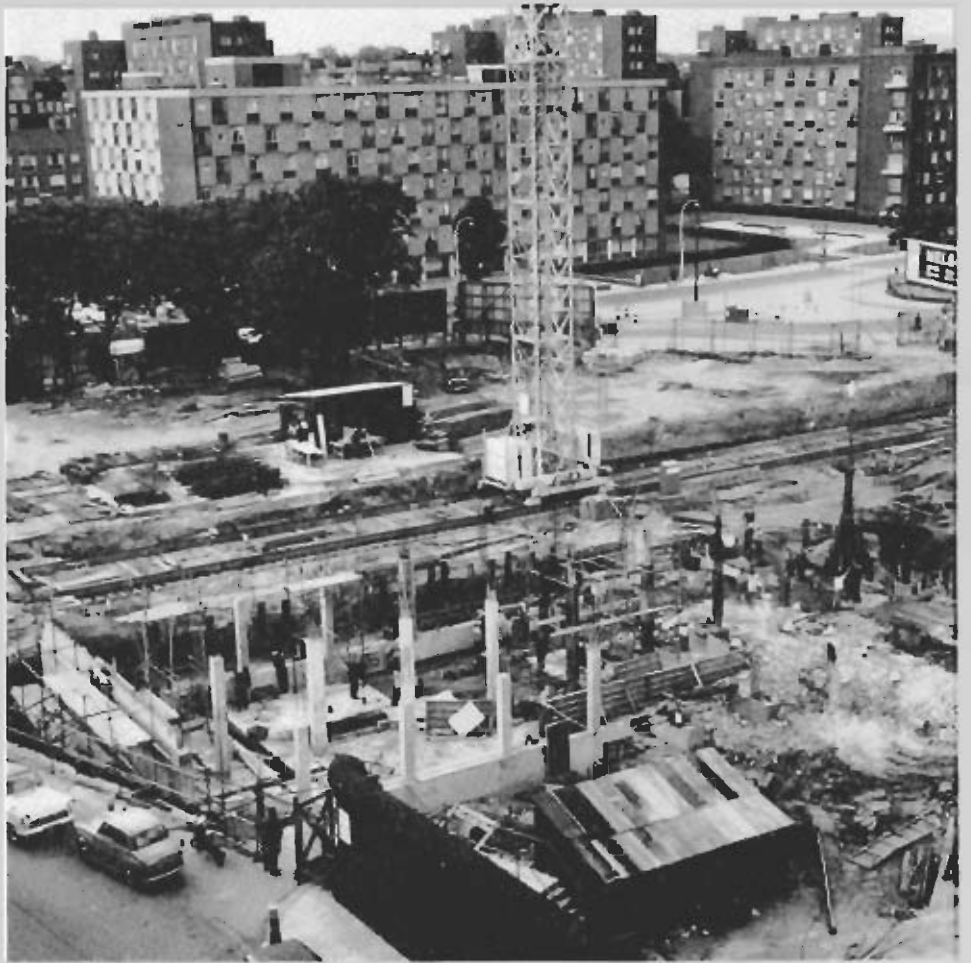
Foundations being laid for new signal box July 1963
