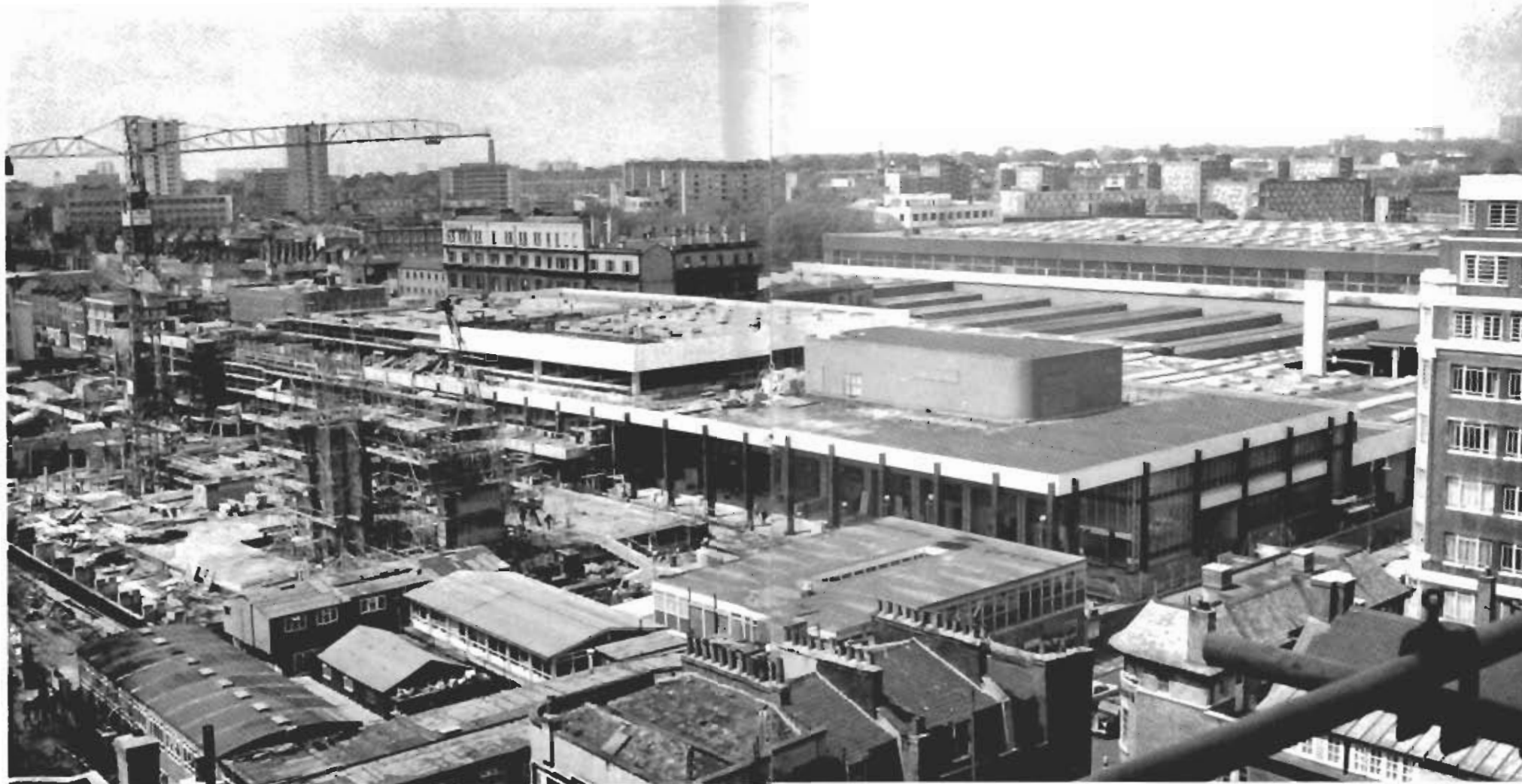
Nearing completion: panoramic view of Station with East Colonnade on right
