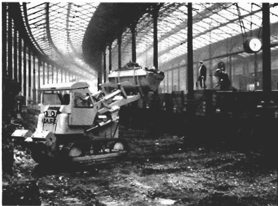
Work starts on new platform. February 1963
