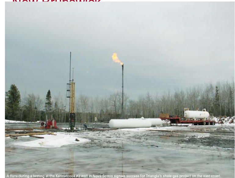
A flare during a testing at the Kennetcook #2 well in Nova Scotia signals success for Triangle's shale gas project on the east coast.
