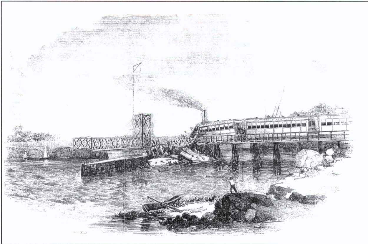
Figure 1.—Originally entitled “The Catastrophe,” the illustration depicts the accident site at the drawbridge with a portion of one passenger car assumed to be the one in which Dr. Russell was riding. The engine struck the abutment followed by a baggage car, two mail cars, and two and one half passenger cars.
