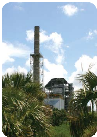
Biomass-fired BFB boiler
