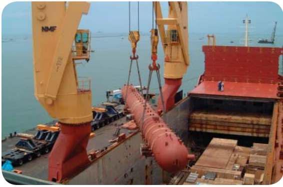
Design for constructability
