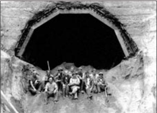
Construction workers at the north portal of the Tawa Flat deviation no.2 tunnel, Glenside c.1930. (Murray J. Henderson Collection, Glenside Progressive Assn. Inc.)
