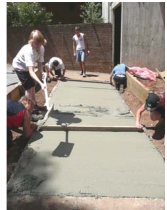
Screeding the surface
