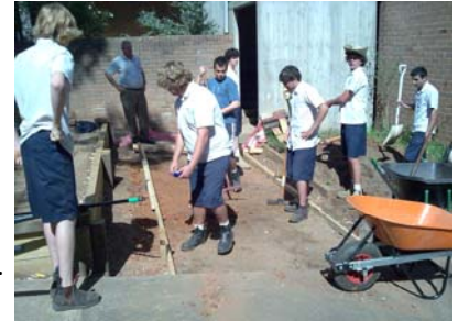
Constructing the formwork for the concrete path
