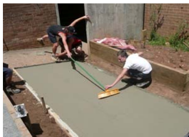
Applying the finishing touches
