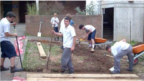
Clearing the delivery area
