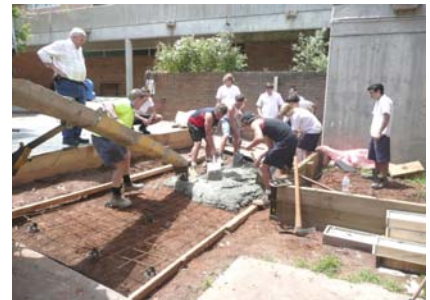
Pouring the concrete
