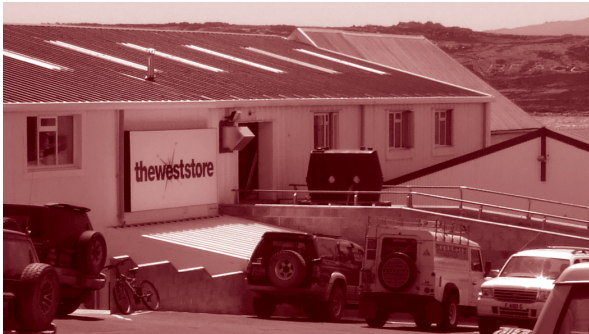
Rear entrance to the extended West Store.
