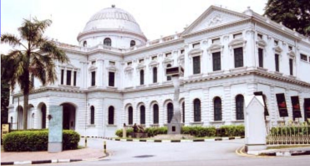
The grand old dame at Stamford Road will be closed for redevelopment in late April 2003.
