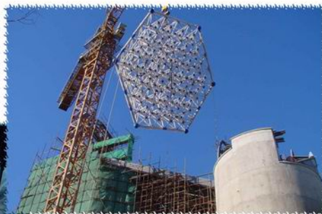
M_B 桁架吊装 Gross mirror cell of M_B during installation
