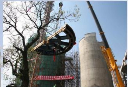
LAMOST项目望远镜开始安装 The installation of the first large parts
