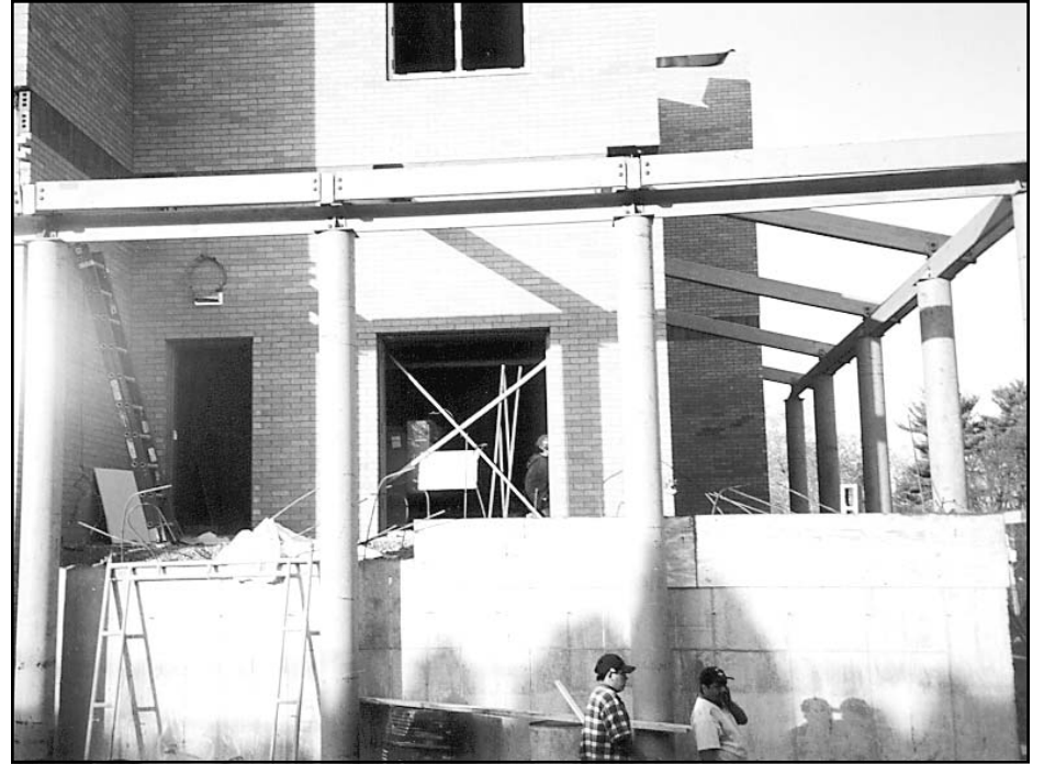
Construction is well underway at Blind Brook's new Middle School.
