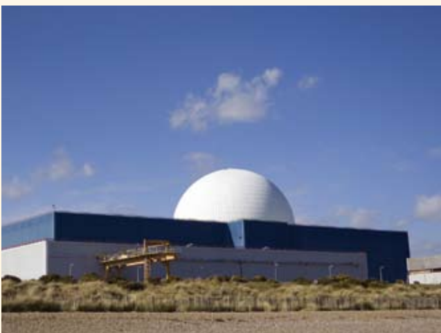
▲ The white dome of British Energy's Sizewell B nuclear power station in Suffolk, U.K., houses a pressurized water reactor.
