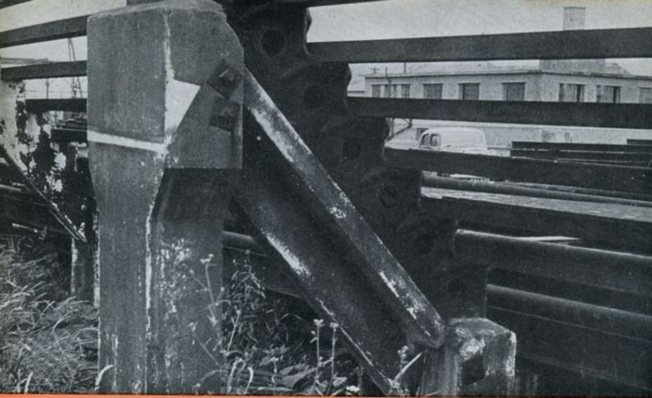
STORAGE RACKS FOR HANDLING THE 4,000 FT. LENGTHS OF 3 IN. PIPE FOR "PLUTO"
