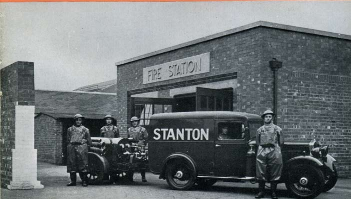
TRAILER PUMP OUTSIDE THE FIRE STATION AT STANTON
