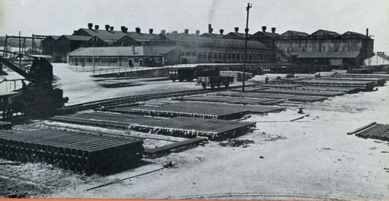
MACHINE SHOP (DALE SPUN IRON PIPE PLANT)
