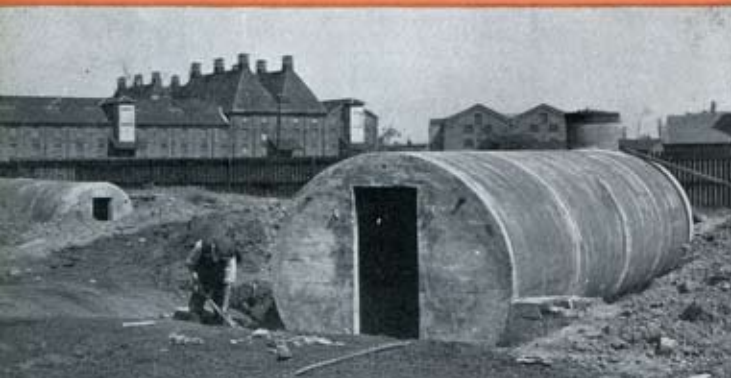
A TUBULAR SHELTER COMPLETED AND IN POSITION
