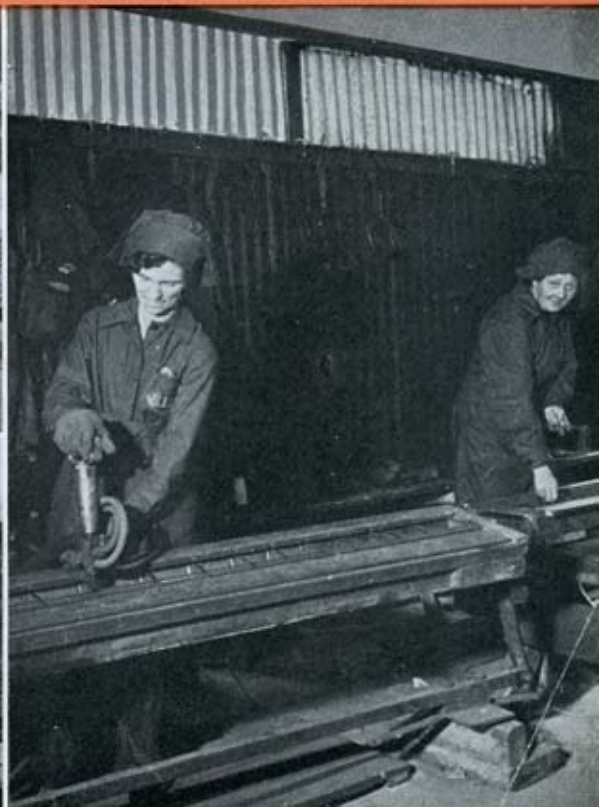
WELDING FRAMES FOR CONCRETE SLEEPERS
