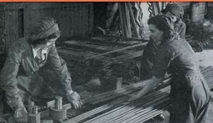
BENDING STEEL RODS BY MACHINERY VIEW OF WELDING SHOP
