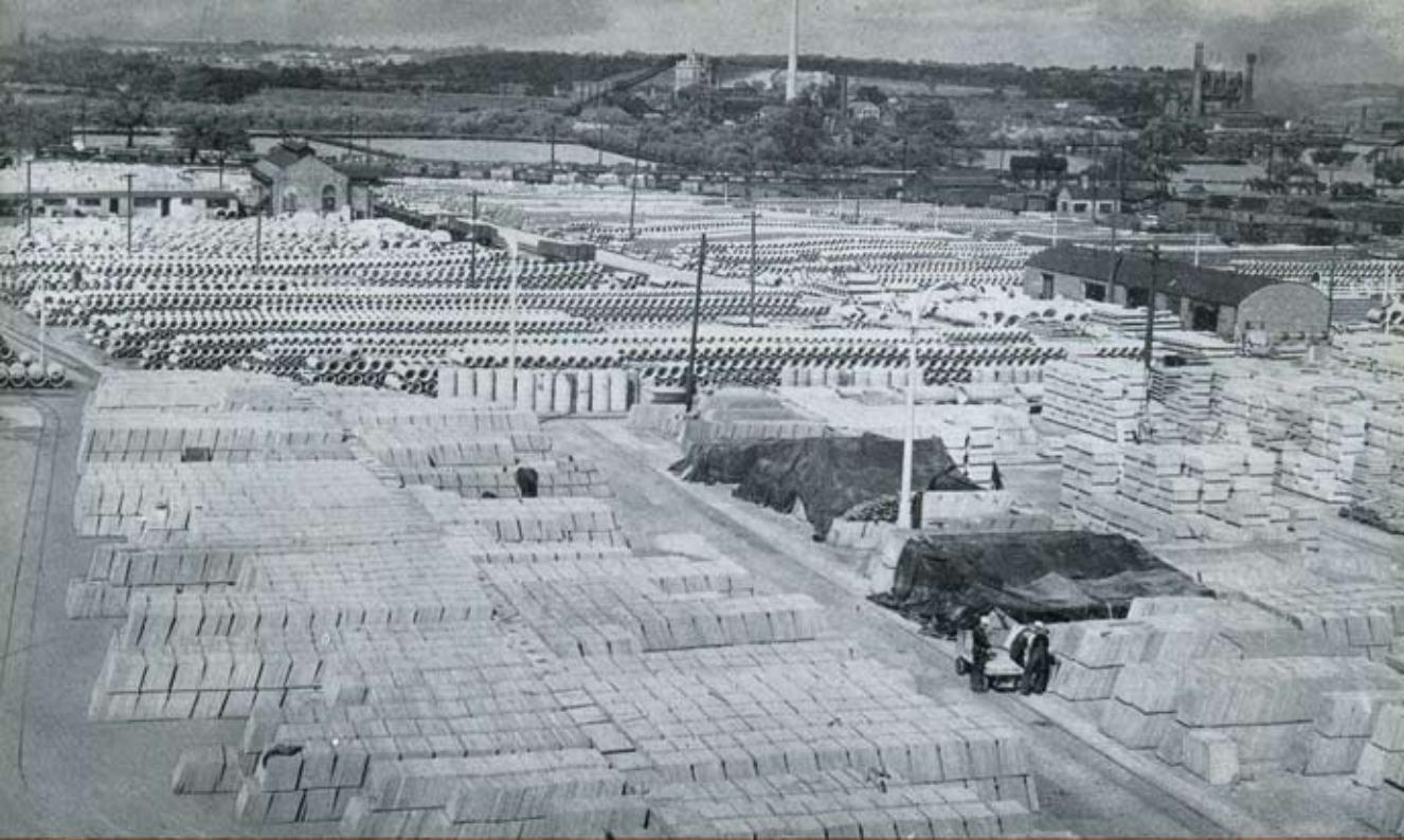
BIRD'S EYE VIEW OF THE CONCRETE PLANT STOCK YARDS
