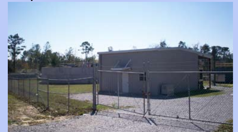
Figure B-59. West Harrison wastewater treatment facility.
