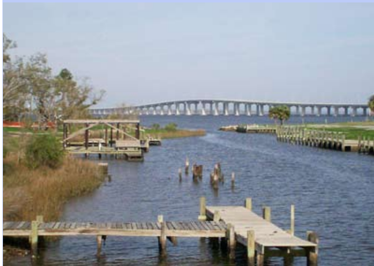
Figure B-48. The new US Highway 90 bridge over the Bay of Saint Louis.
