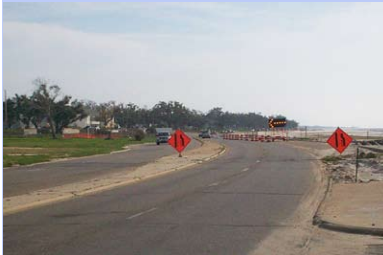
Figure B-47. Construction continues along US Highway 90.
