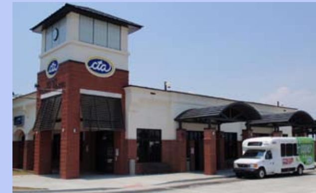
Figure B-52. The new Biloxi transit center.
