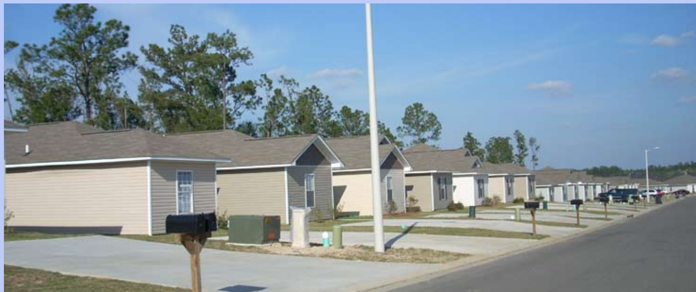
Figure B-18. Quail Creek is an example of a subdivision with townhome-style residential units that will be served by water and sewer.
