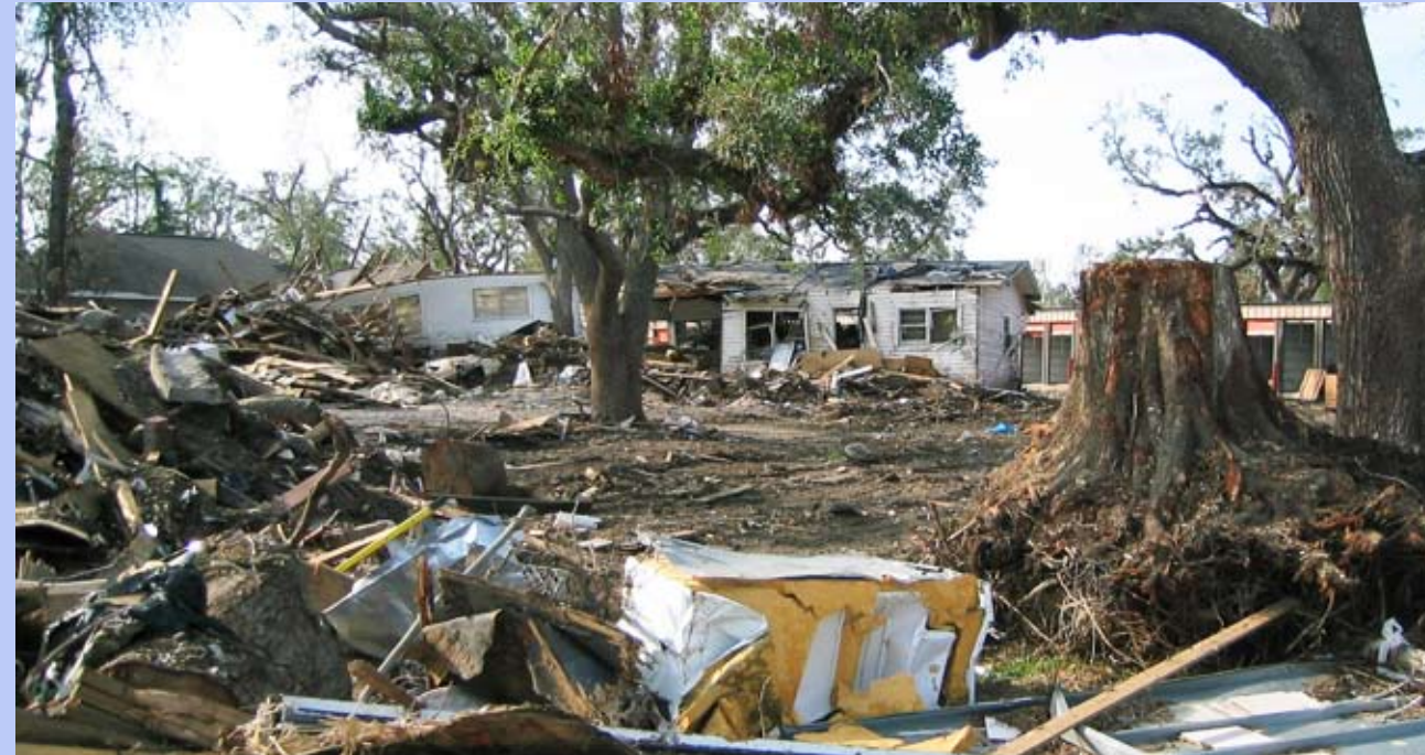
Figure B-42. Hurricane Katrina caused catastrophic damage.
