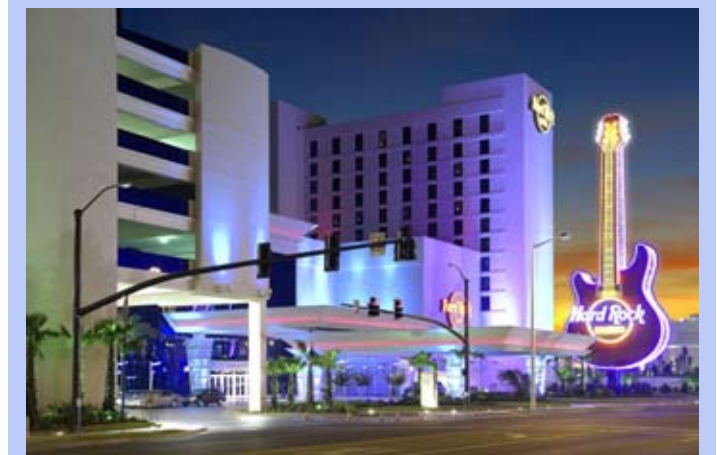
Figure B-12. The Hard Rock Casino is one of nine casinos located in Harrison County in 2008.
