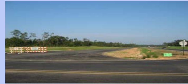
Figure B-51. State Highway 67 is currently under construction.
