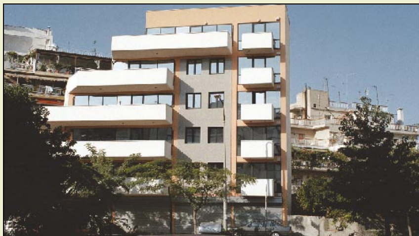
The building that houses the Research Committee in K. Karamanli street (N. Egnatia).
