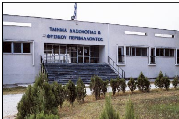
Facilities of the School of Forestry and Natural Environment in Finikas, Thessaloniki.
