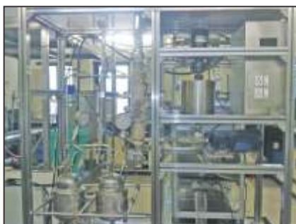
Continuous Pretreatment Pilot Plant
