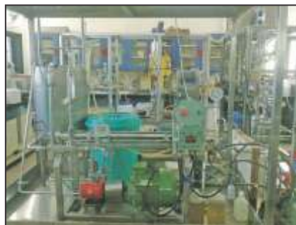
Pilot Plant Assembly (Nanofiltration)
