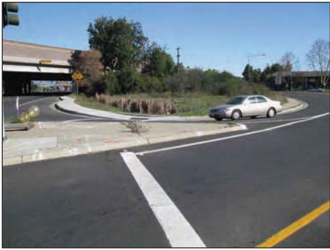
Pork-chop islands can be problematic for bicycles due to odd angles and high speed traffic.
