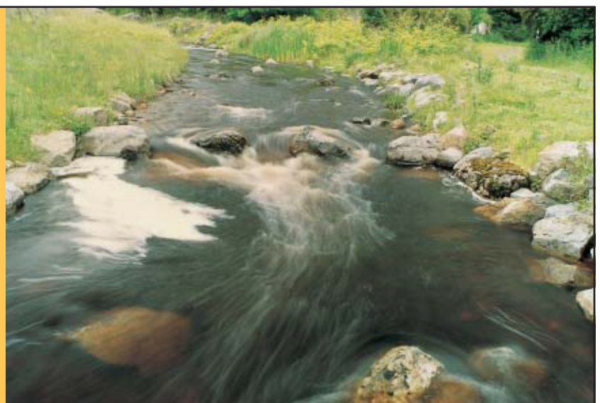
A vortex rock weir concentrates the flow to the centre of the pool, creating depth and providing cover.
