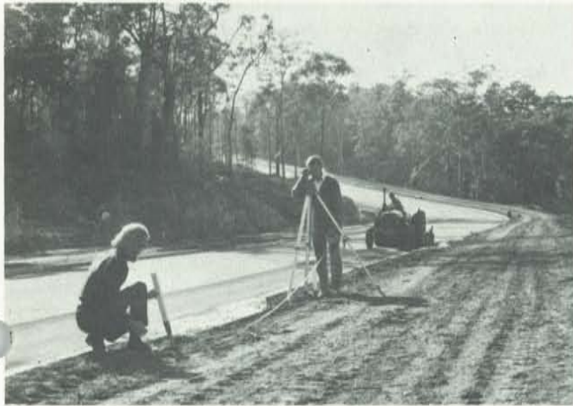
New road almost completed through what was once a deep gully.
