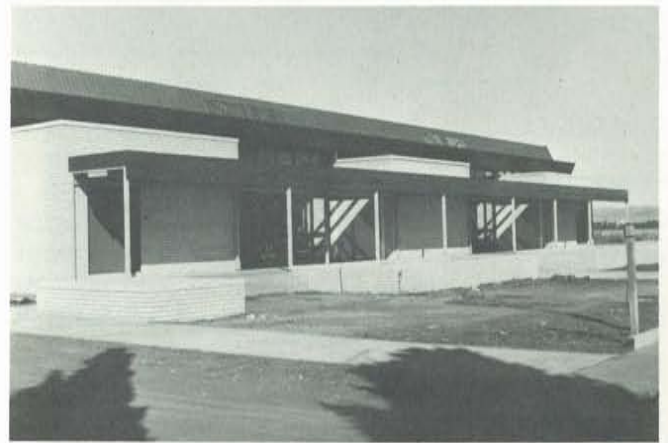
Front view of building.
