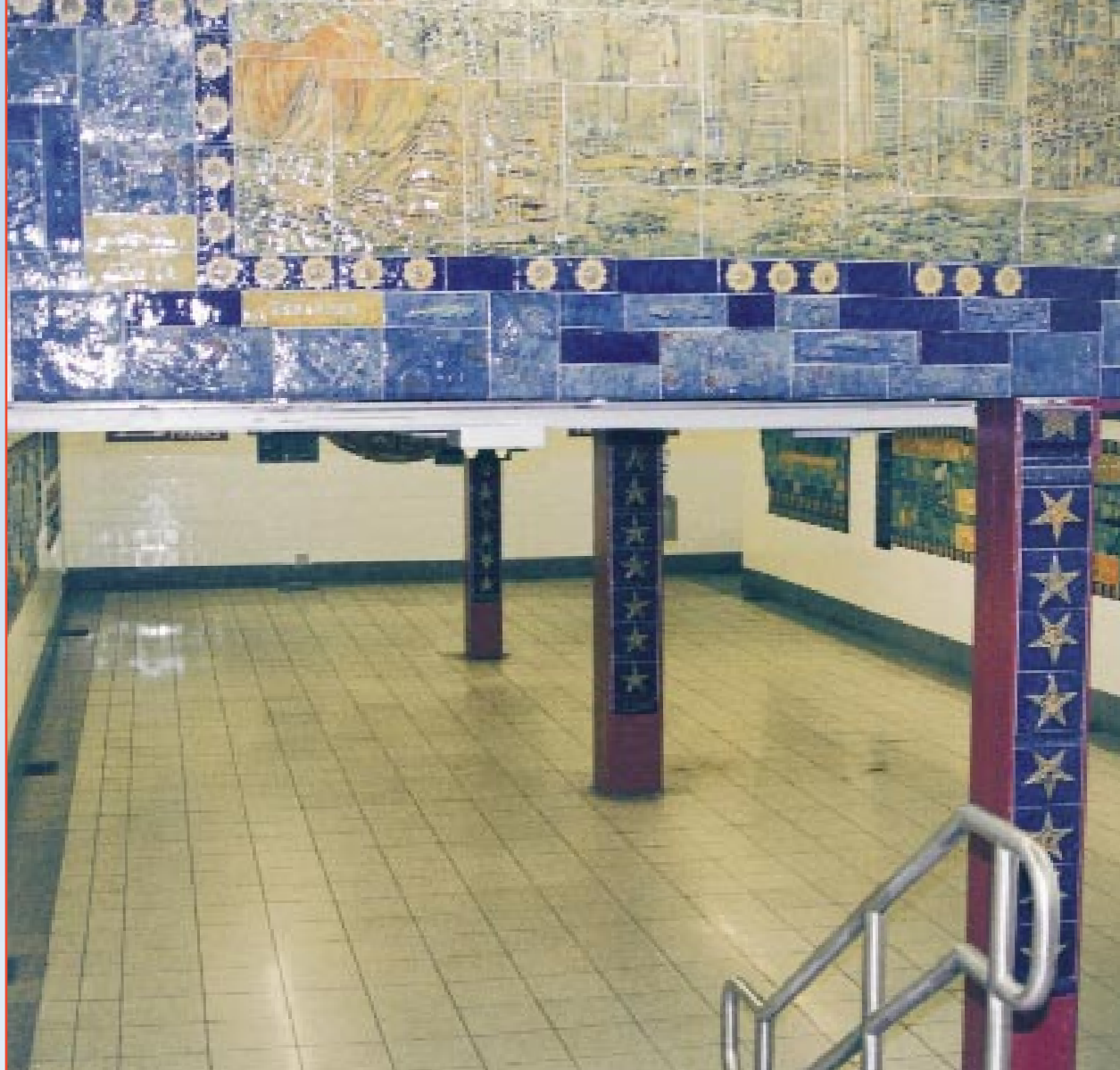
TSM #3 introduces a new passenger walkway from Fulton Street IRT station to the World Trade Center concourse.
