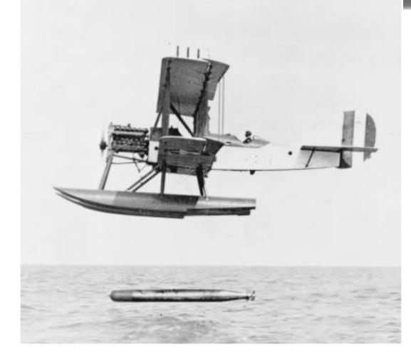
Launching torpedo from R-type aircraft, a means of increasing Naval aviation's offensive power 1061481
