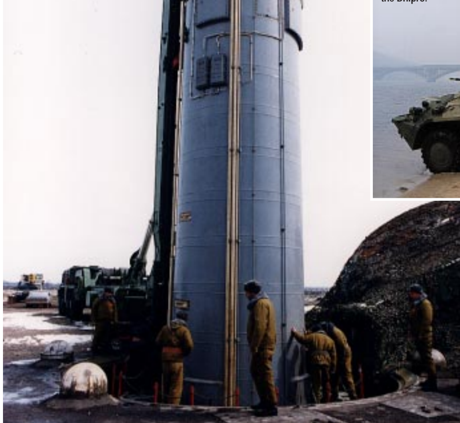
Removing SS-19 missile from silo.
