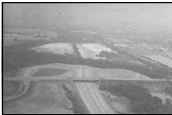
Aerial view of the I-670 stub before construction. Sludge lagoons are visible towards the top of the photo.
