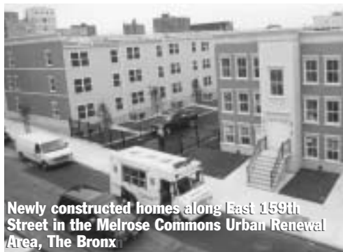
East 159th Street in the Melrose Commons Urban Renewal Area, The Bronx
