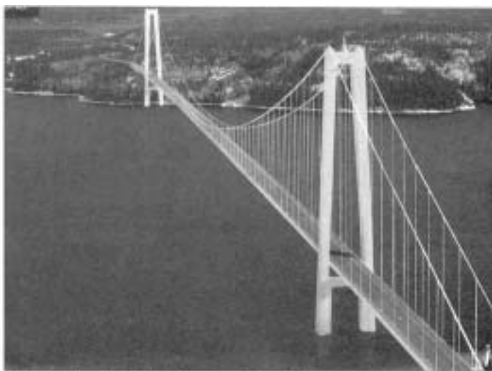
34. Høga Kusten Bridge, Sweden, 8th with respect to span length at the change of the millennium. PHOTO VÄGVERKET REGION MITT
