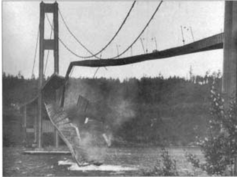
Fig. The first Tacoma Bridge
