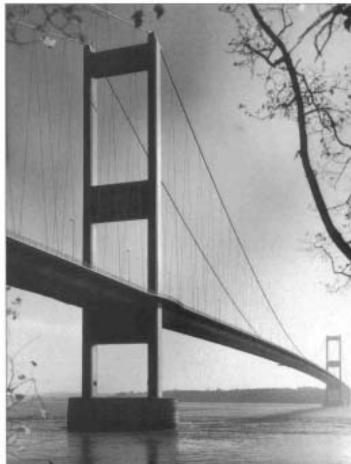
26. Severn Bridge, Britain, the first major suspension bridge to have both a streamlined steel box girder deck and inclined hangers. PHOTO BRITISH ROPES LTD
