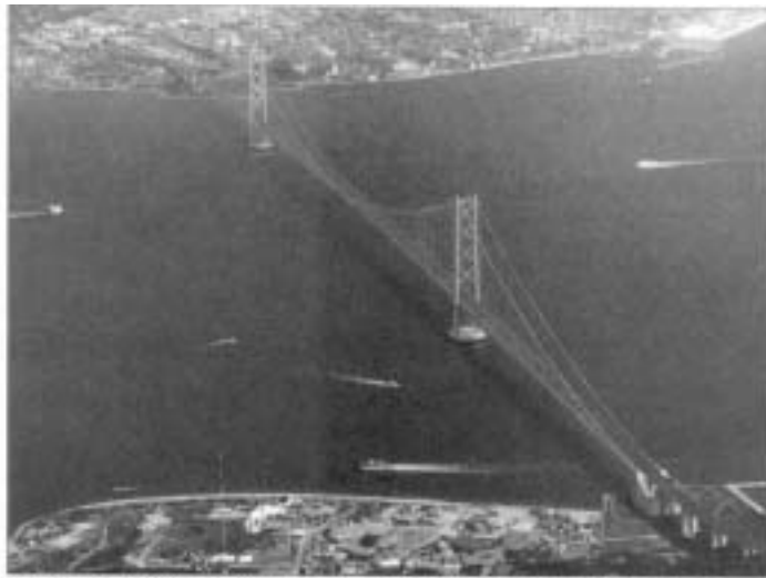
39. Akashi-Kaikyo Bridge, Japan, record bridge in many respects, among them the longest main span of any bridges. PHOTO HONSHU-SHIKOKU BRIDGE AUTHORITY
