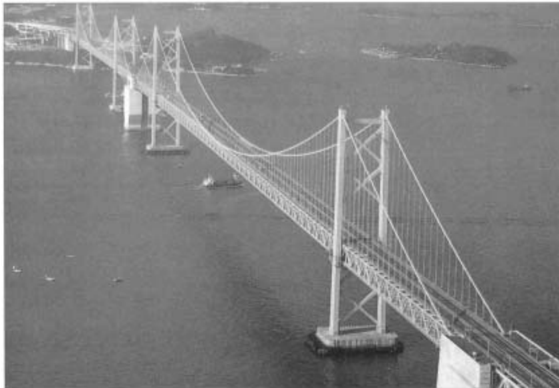
33. Seto-Ohashi succession of bridges, Japan, currently the world's longest highway/railway bridge. PHOTO HONSHU-SHIKOKU BRIDGE AUTHORITY
