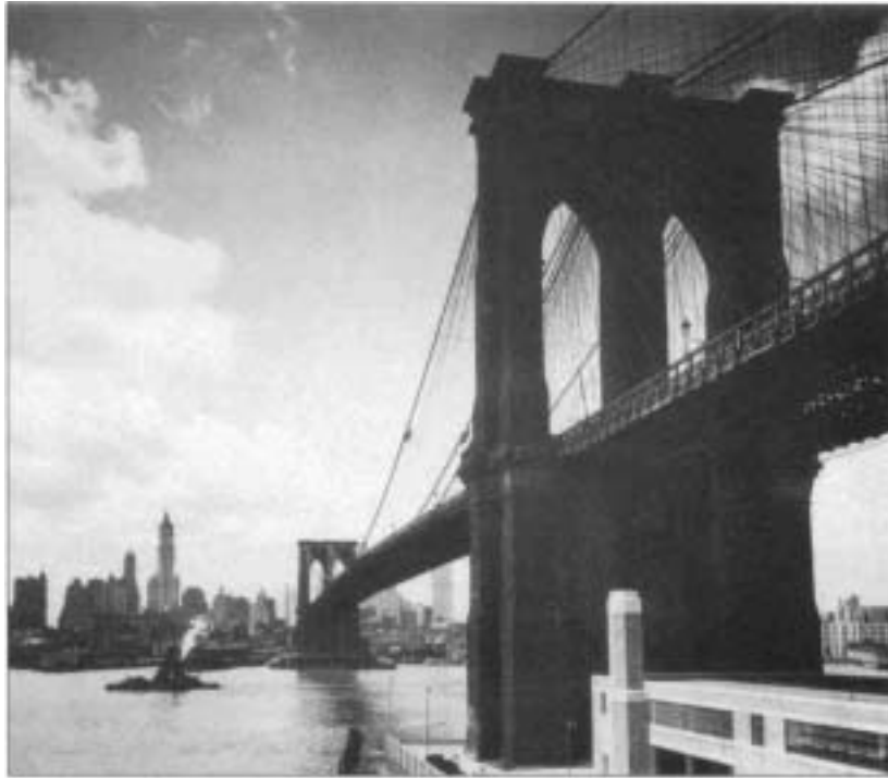
Fig. Brooklyn Bridge
