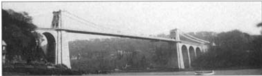
Fig. Menai Bridge
