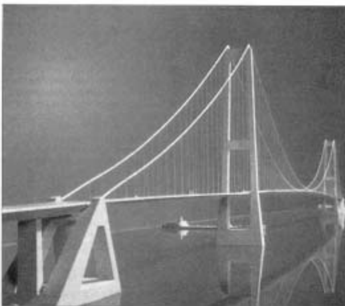
35. Great Belt Bridge, Denmark, for a short period the world's longest-span suspension bridge. PHOTO STOREBÆLTSFORBINDELSEN
