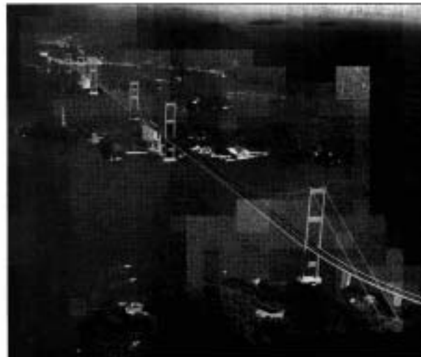
38. Kurushima Bridges, Japan, a rare construction of three successive suspension bridges with two shared cable anchorages. PHOTO HONSHU-SHYOKU BRIDGE AUTHORITY
