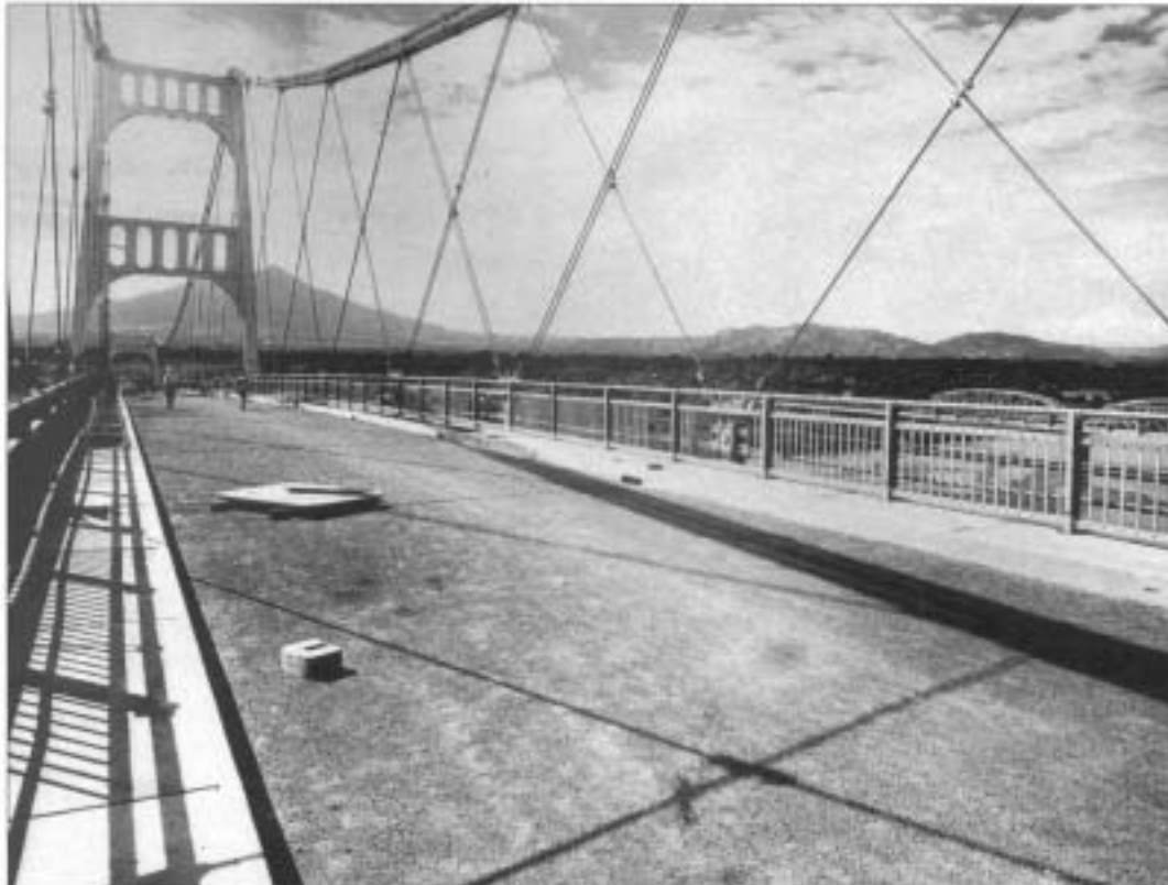
28. San Marcos Bridge, El Salvador, a rare feature of criss-cross hangers.
