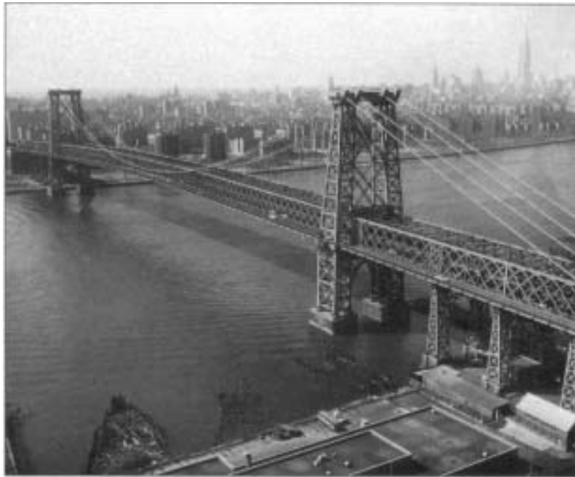
Fig. Williamsburg Bridge, New York City
