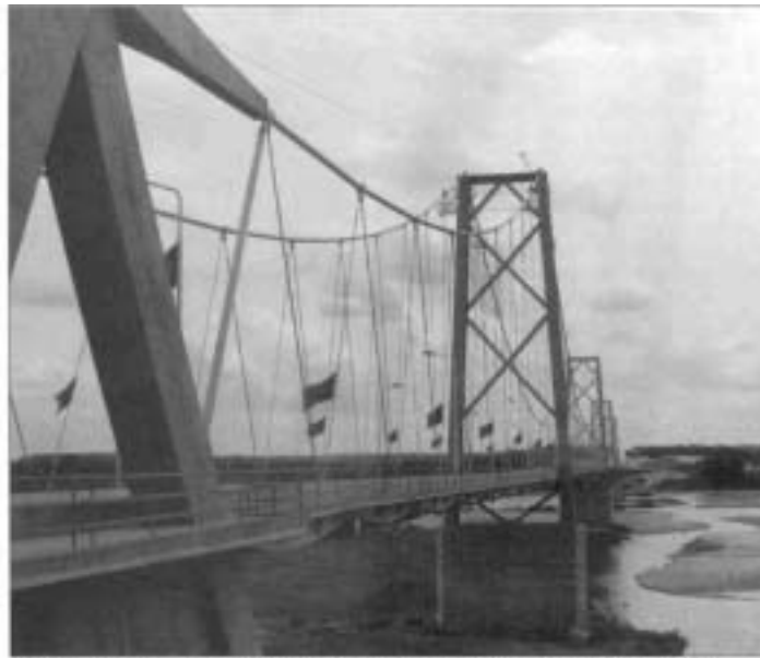
27. Save Bridge, Mozambique, five successive suspension spans, concrete deck structure, and inclined hangers.
