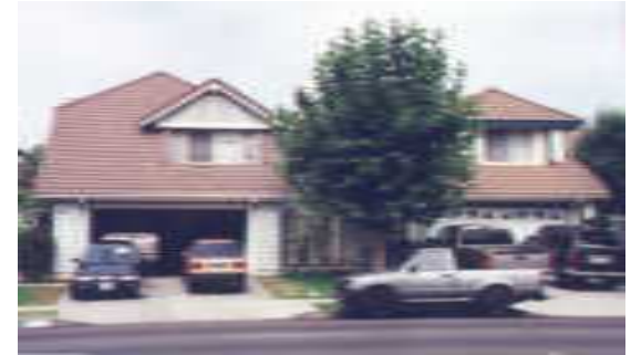
Image 17: High density is also prevalent in recently built homes.
