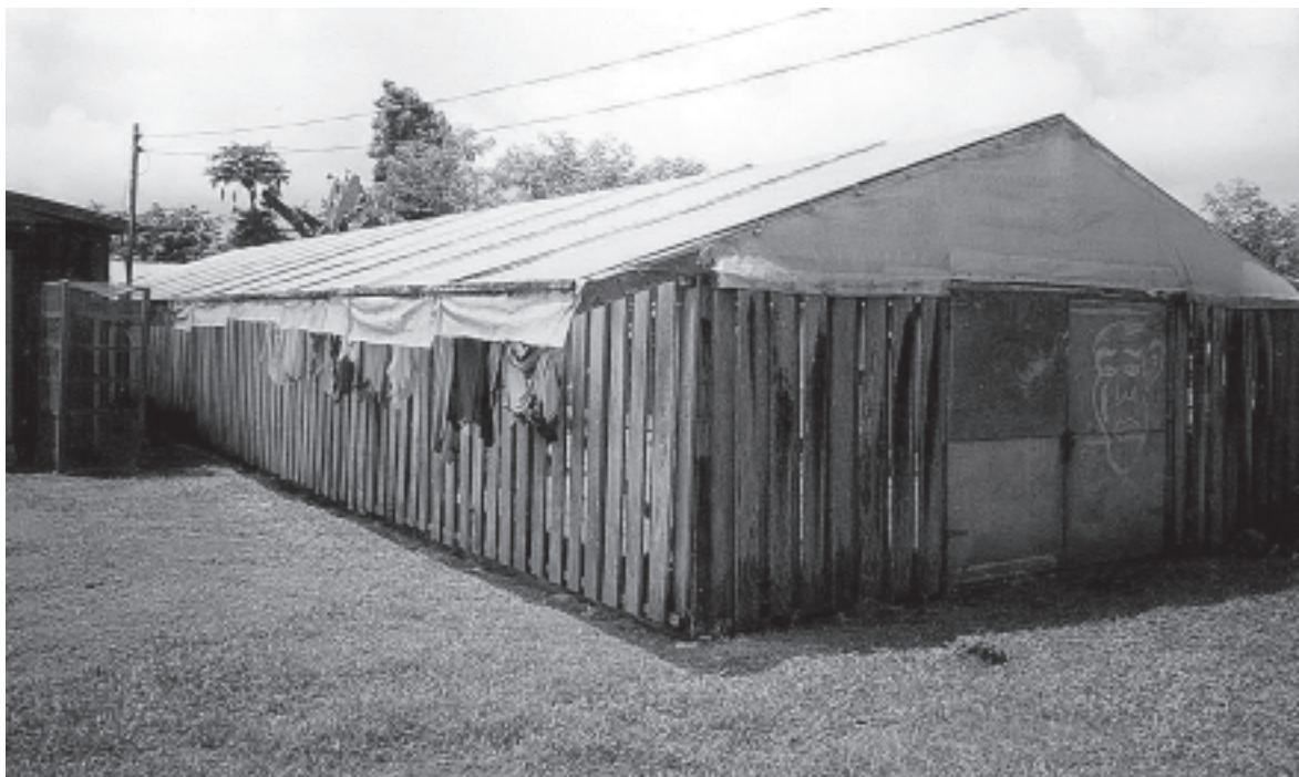
A kava drying shed in Samoa with clear plastic roof and vents on sides.
