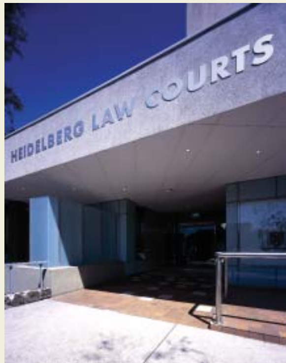
Exterior view of Heidelberg Law Courts. A $4.8 million extension and refurbishment of the court was completed in August 2002.
